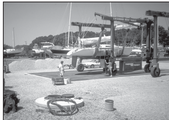
Figure 4-11. Lockwood Boat Works (New Jersey) regraded its combined parking and boat maintenance yard and surfaced it with 6 inches of crushed concrete to successfully control runoff. Using recycled concrete crushed into stone-sized pieces, the cost was $18,000 per acre installed, whereas crushed rock would have cost $27,000 per acre and asphalt paving would have cost $54,000 per acre (USEPA, 1996: Clean Marinas—Clear Value ).
