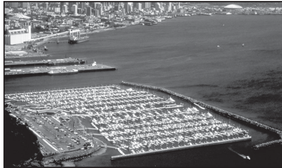
Figure 4-6. Habitat assessment was used at Elliot Bay Marina (Washington) to design the marina to work with natural habitat function. Wide openings between rock groin-type breakwaters, docks, and beach give easy access to migrating juvenile salmon leaving Puget Sound, while providing good water circulation and tidal changes inside the marina basin. A man-made 1,500-foot-long sandy beach has replaced lost habitat, providing a feeding ground for young salmon. Schools of young salmon and herring move throughout the marina basin (USEPA, 1996: Clean Marinas—Clear Value ).
