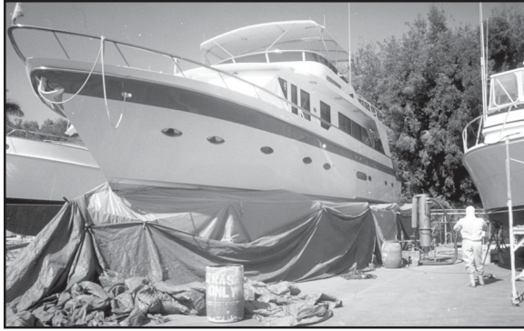
Figure 4-17. Associated Marine Technologies (Florida) took prevention of hull sand-blasting debris a step further by switching from a silica wet/dry sandblasting medium to a closed system that employs a reusable plastic material. The facility uses a high-capacity plastic-medium-blasting dry stripper and a media reclaimer that recovers the plastic material and separates it from the paint dust. This process significantly reduces the cost of cleanup and disposal, gives a higher-quality surface, and is much less aggressive on the gelcoats of fiberglass hulls (USEPA, 1996: Clean Marinas—Clear Value )
