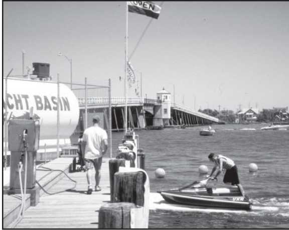
Figure 4-13. Two PWC floating docks were installed at Winter Yacht Basin, Inc. (New Jersey). The floats are 4 feet by 10.5 feet and are connected to PVC pipes to allow them to ride up and down with the tide. Operators of PWCs can drive up onto the platform, step off, and fill the tank from the dock. The platform is stable enough to limit spilling during fueling. This practice has also decreased conflict between PWCs and larger boats at the fuel dock and has increased fuel sales at the marina (USEPA, 1996: Clean Marinas—Clear Value ).
