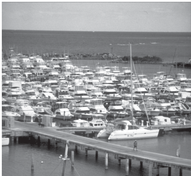
Figure 4-2. Puerto Del Ray Marina (Puerto Rico) has an offshore rubble mound breakwater that protects the southeastern and eastern exposures of the marina. Two hundred feet of the southern breakwater was removed, creating a new south side breachway exit/entrance that is still well protected but now allows for greater circulation in the basin. Water clarity improved after the alteration, and as a result new customers (a 3 percent increase for the marina) relocated to Puerto Del Rey Marina (USEPA, 1996: Clean Marinas—Clear Value ).
